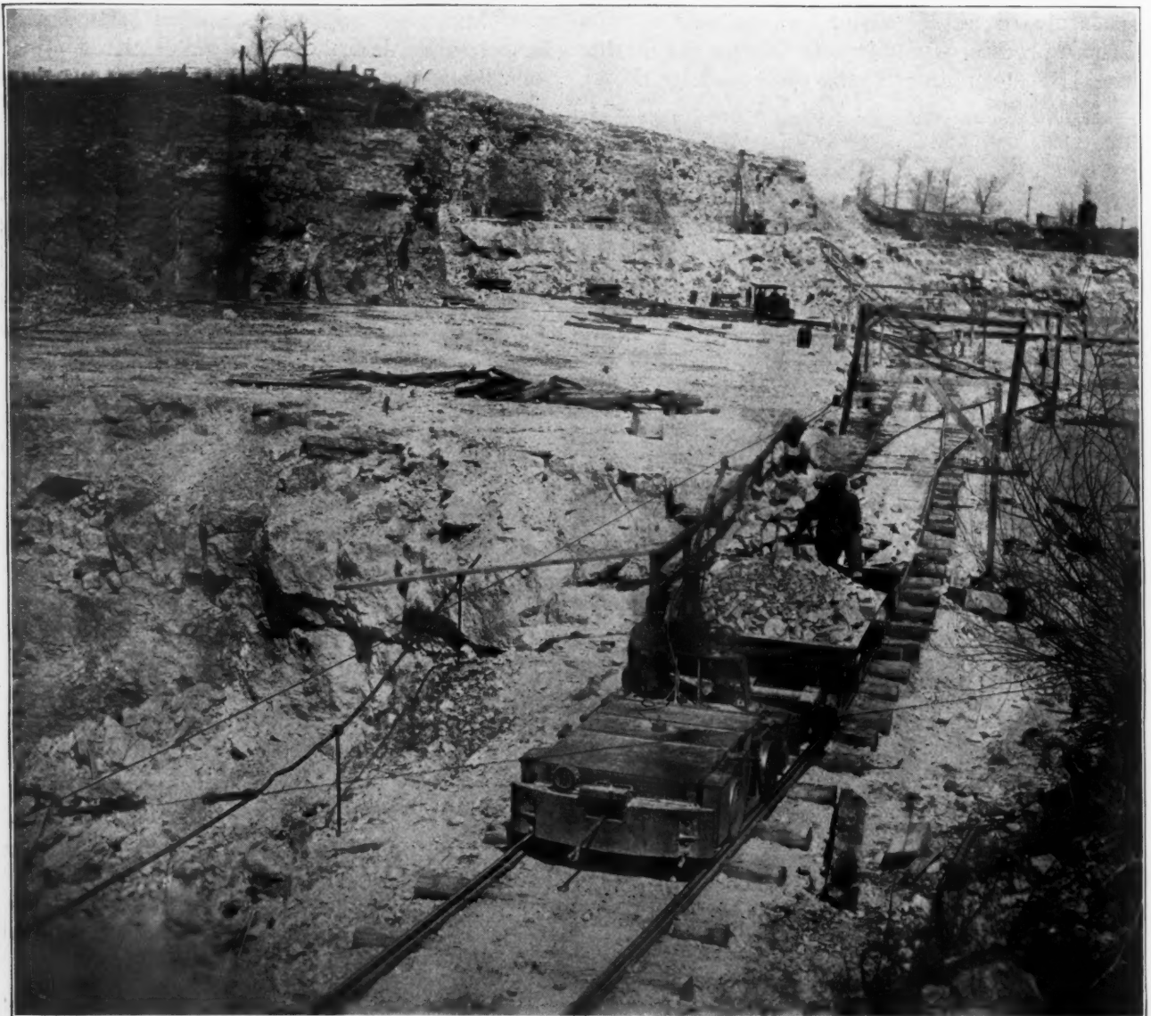
Electric Locomotive Conveying Material to Crushers
